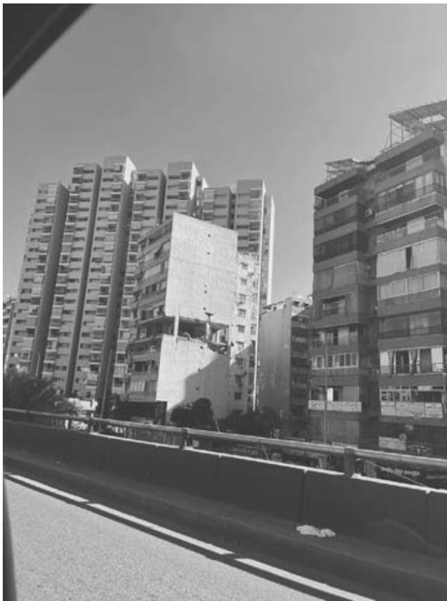
Fig. 1 A building, targeted by the IDF, viewed from the highway from the airport towards the city centre
