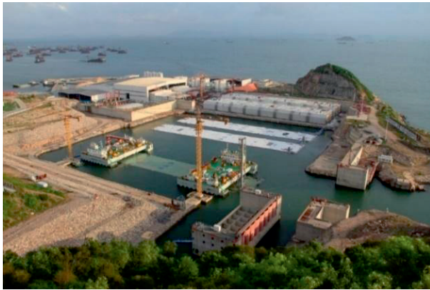
(a) HZMB link immersed tunnel factory (b) factory conceptual layout for mega shelter
