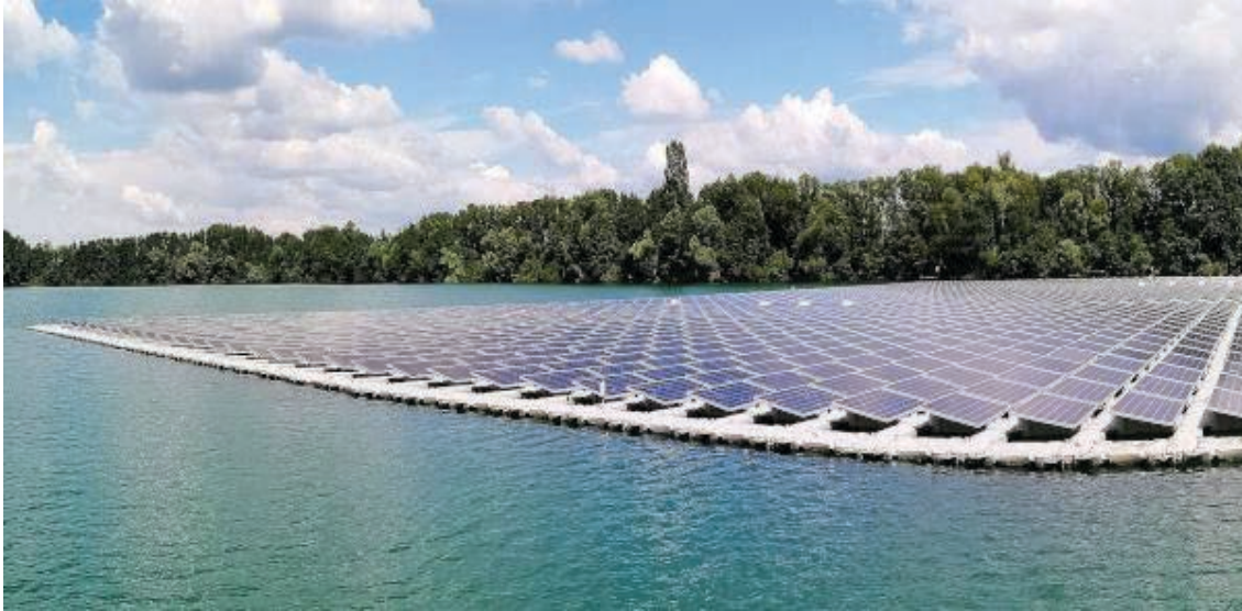
Fig. 1: Floating photovoltaic plant on a gravel pit lake in south-western Germany (photo: Fraunhofer ISE).
