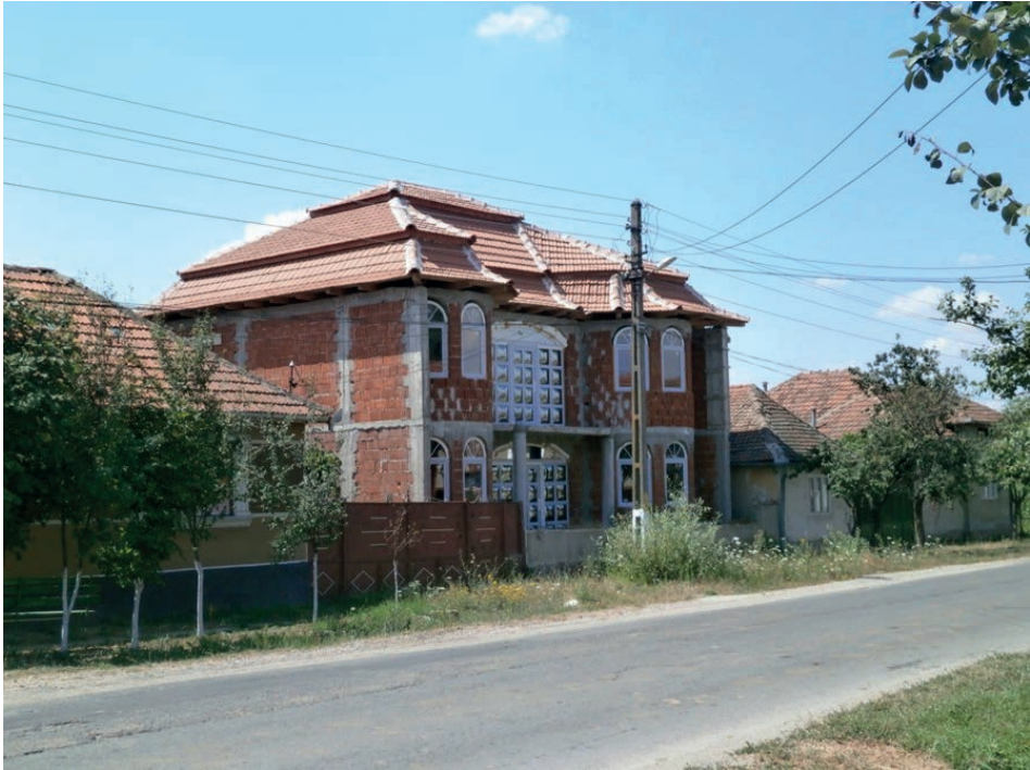
10. Ucuriș, house in the making, main road
