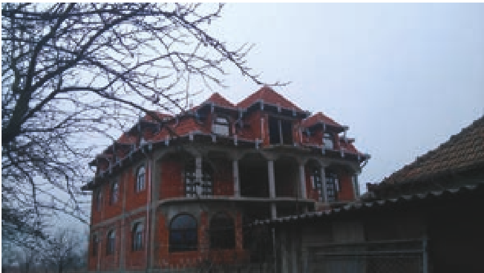
11. Ucuriș, house in the making, side road
