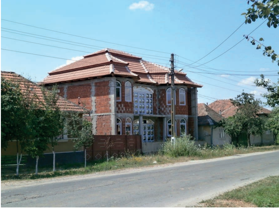
10. Ucuriș, house in the making, main road
